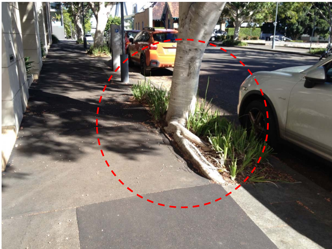
Photo 2: Displacement of kerbs due to roots of existing juvenile trees.
