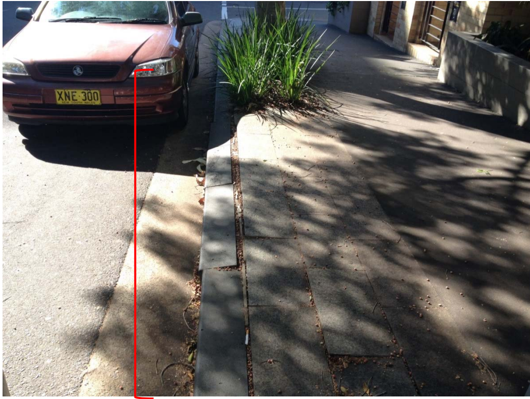
Photo 2: Displacement of kerbs due to roots of existing juvenile trees.
