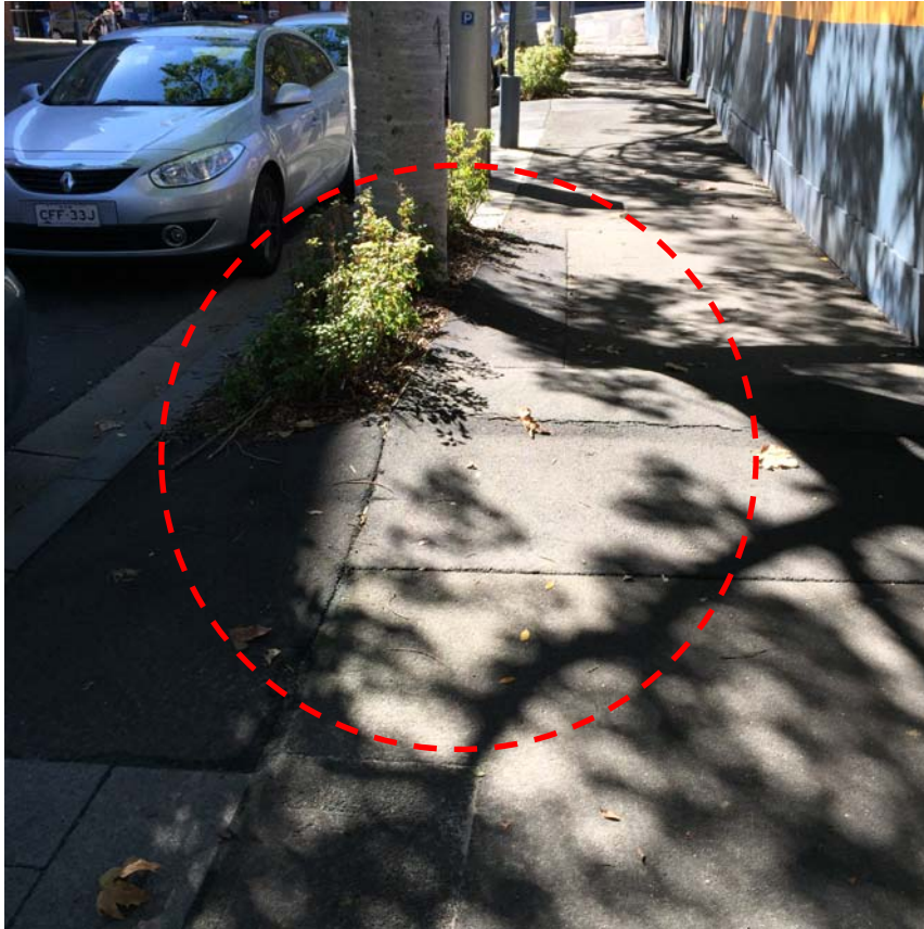
Photo 6: lifted asphalt paving
