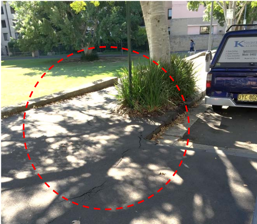
Photo 6: lifted asphalt paving
