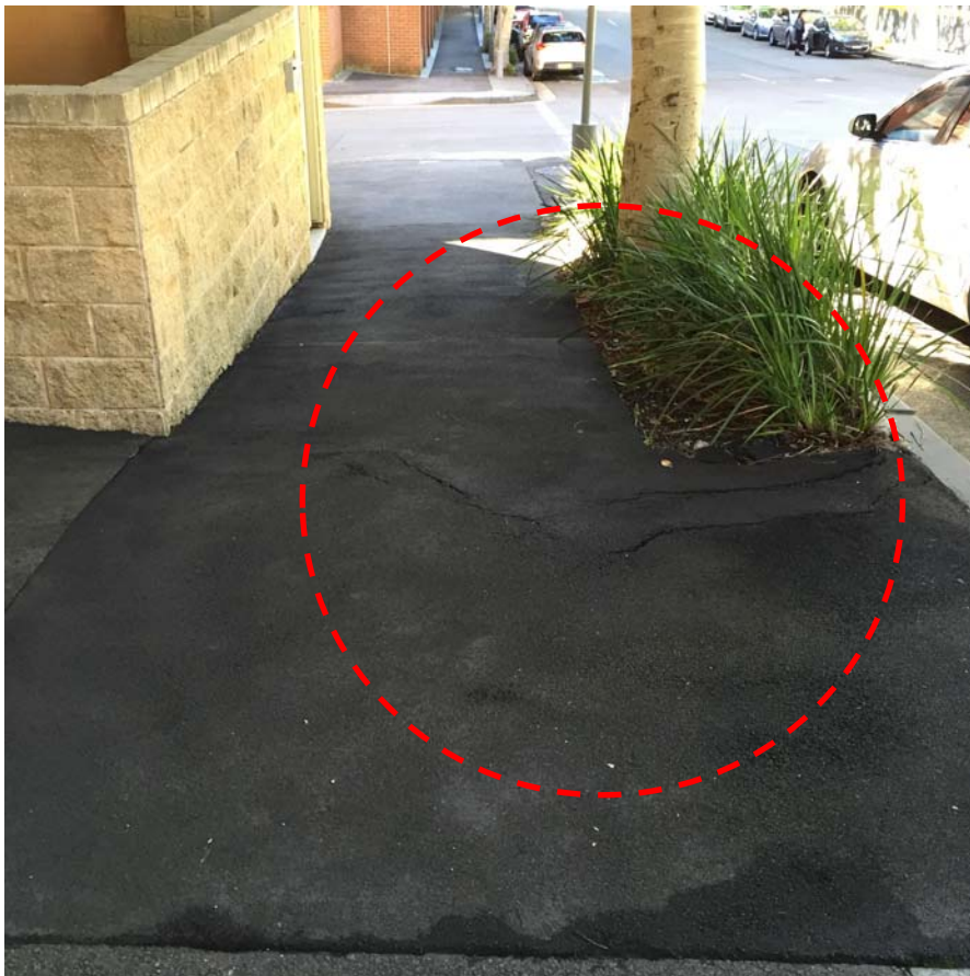
Photo 4: lifted asphalt paving
