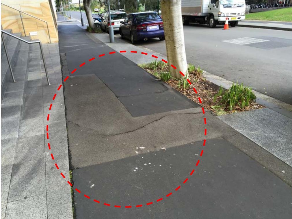
Photo 4: lifted asphalt paving
